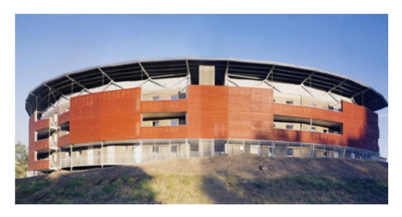
Low cost modular flats in Leeds: built 2000, demolished 2005 owing to concerns over stability in strong winds.
