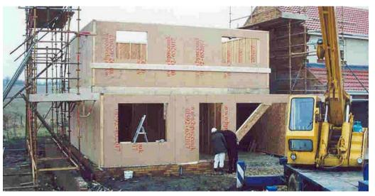
SIPs – structural insulation panels
