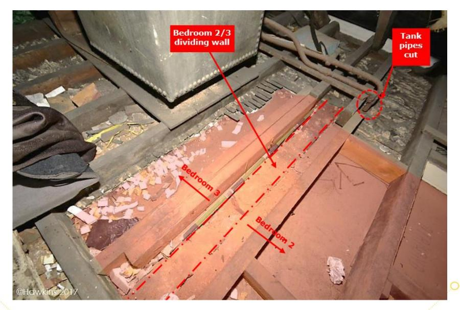
Lath and plaster ceiling to rear of tanks replaced
